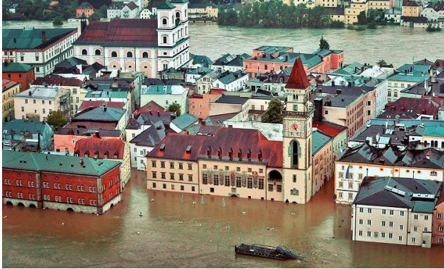
Floods in Germany June 2013, damage 3 billion € - insurance claims
